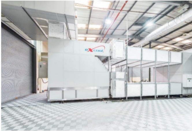
The “Excool” Indirect Evaporative Data Centre Cooling unit
