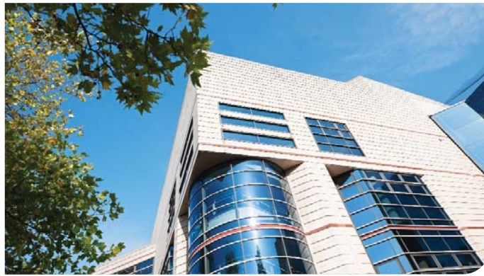
Birmingham's International Convention Centre benefited hugely from the commissioning manager being responsible to the main contractor and adequate time and budget allowed for the commissioning.
