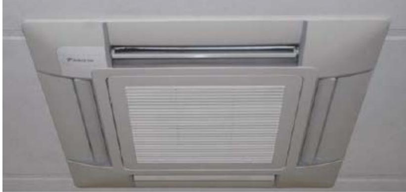
Figure 4 Ceiling mounted cassette unit DX System
