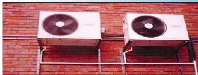
Figure 3 Condenser Units DX split system
